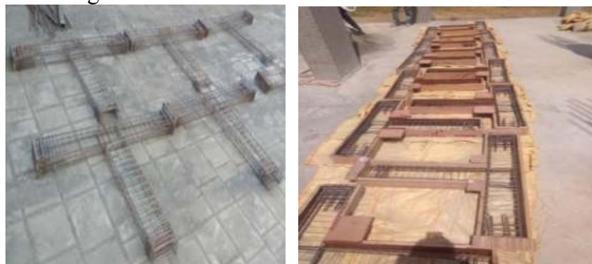
(a) Reinforcement details (b) Form work for casting Fig. 3: Reinforcement and Setup for casting
