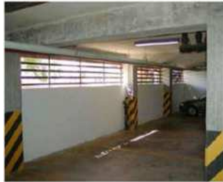
Figure 1.2: Partial infilled wall - short column formed [21]
