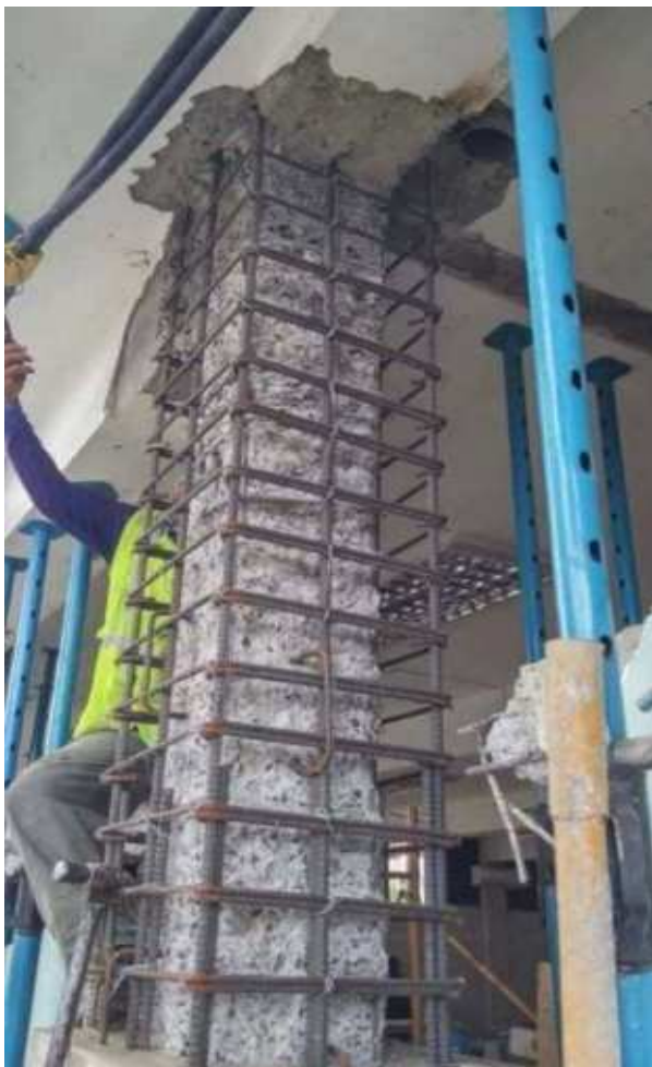
Fig. Retrofitting-for structures by Strengthening
