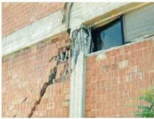
Figure 1.5: Short column failure [2]
