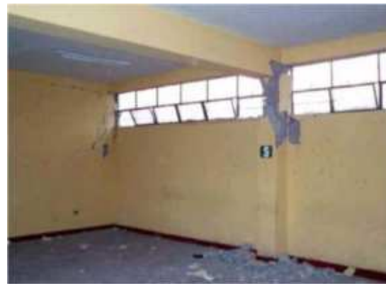
Figure 1.6: Damaged column [3]
