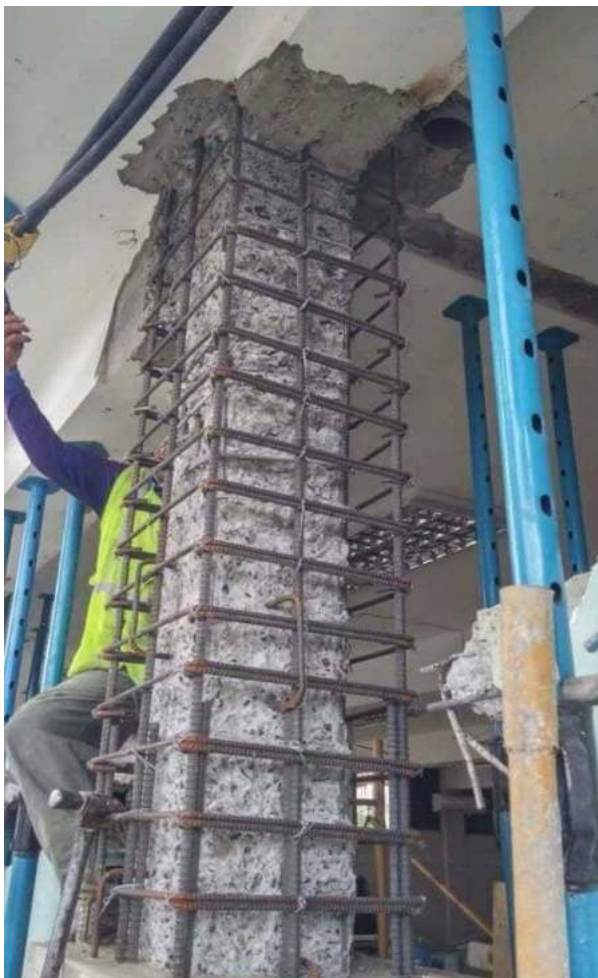
Fig. Retrofitting-for structures by Strengthening
