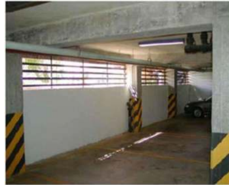
Figure 1.2: Partial infilled wall - short column formed [21]
