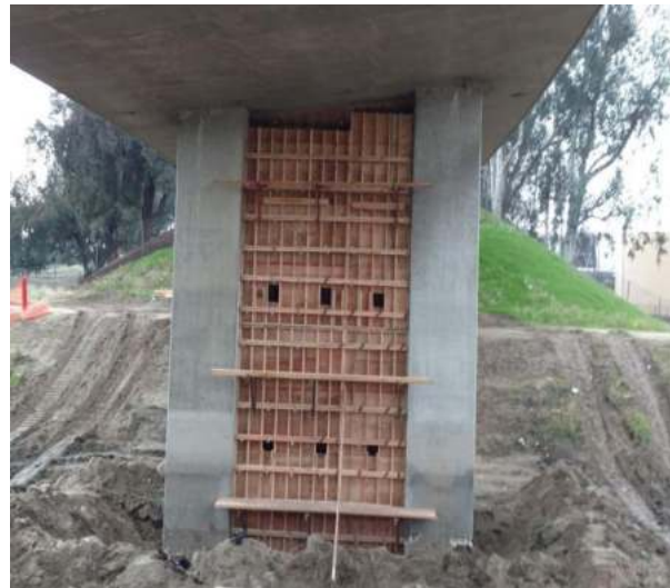
Fig.Retrofitting of a bridge
