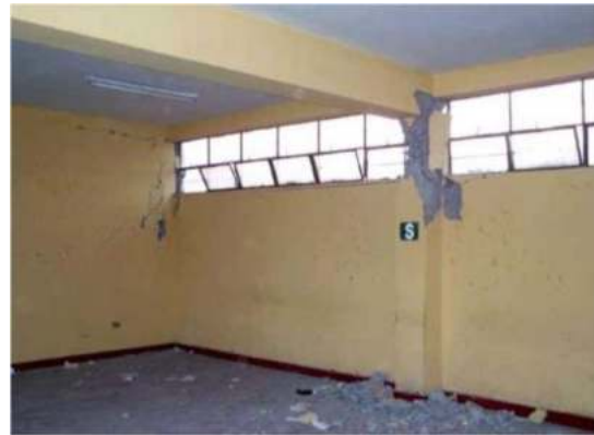
Figure 1.6: Damaged column [3]
