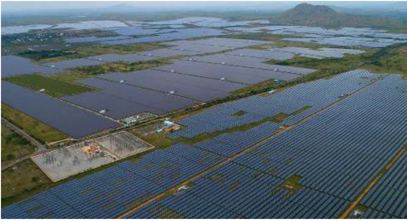
Figure 11(pargada solar plant)
