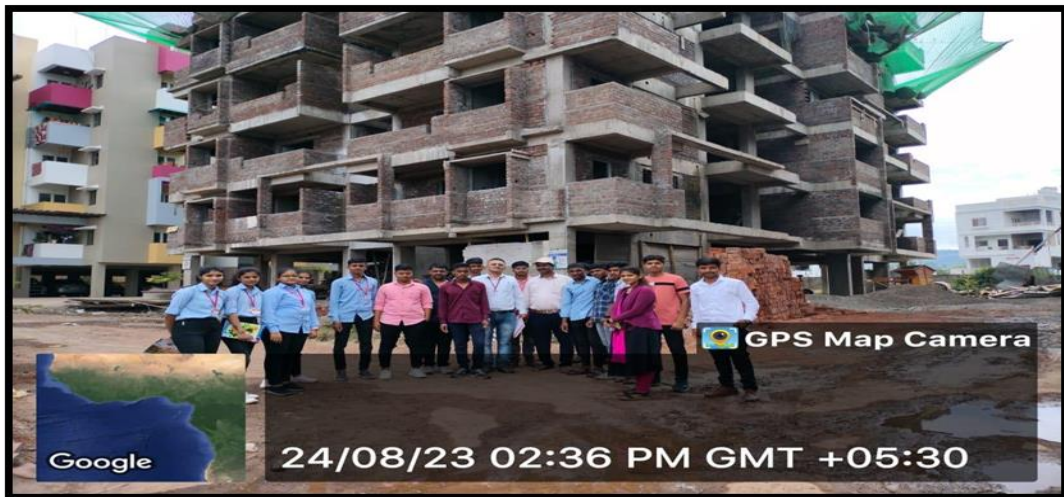
Industrial Visit to Krushnkunj Apartment, RMC plant (Kangralkar Associate) by Mr.Sapkal R.N.
